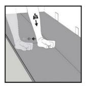
Press down with your hand or tap lightly with a Kährs handblock on the tile you just installed.
