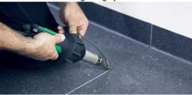
Allow the welding rod to cool slightly before cutting. Use a Mozart knife or moon knife with plate for rough cutting and a Mozart knife or moon knife for fine cutting. Be careful when soldering in fold-ups. The sheet must not be heated too much when folding it up and down, as this can cause damage to the floor.
