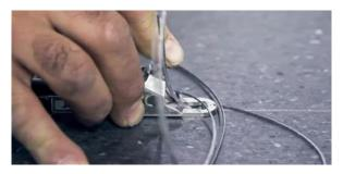
Use a suitable temperature (slightly higher than for PVC) when welding joints and maintain the correct welding speed to avoid changes in the surface protection. Use a welding nozzle with a lip to make good contact between the rod and the sheet. Test heating is highly recommended.
