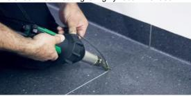
Allow the welding rod to cool slightly before cutting. Use a Mozart knife or moon knife with plate for rough cutting and a Mozart knife or moon knife for fine cutting. Be careful when soldering the Zero in fold-ups. The sheet must not be heated too much when folding it up and down, as this can cause damage to the floor.
