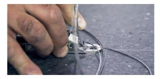
Use a suitable temperature (slightly higher than for PVC) when welding joints and maintain the correct welding speed to avoid changes in the surface protection. Use a welding nozzle with a lip to make good contact between the wire and the sheet. Test heating is highly recommended.
