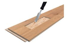
Chisel out the strip and 2 mm of the intermediate layer using a wood chisel.
